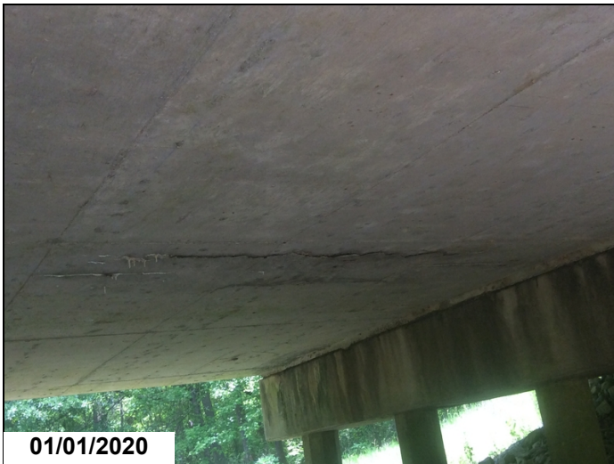
Span soffit Delams.
