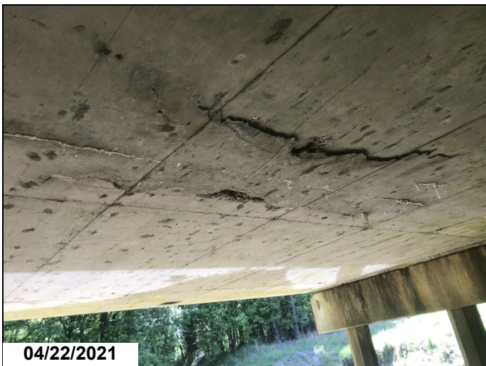
Span 3 soffit delam with staining.
