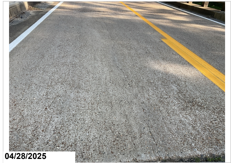
Deck Span 1: Large unsealed cracks.
