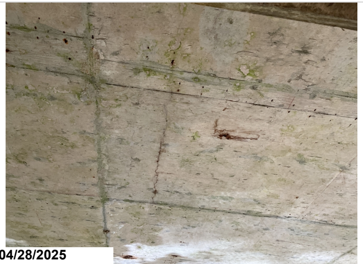
Undersurface Span 2: Large unsealed cracks with staining.
