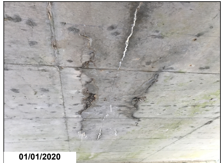
Span 3 longitudinal cracking reflecting thru to soffit with efflorescence.
