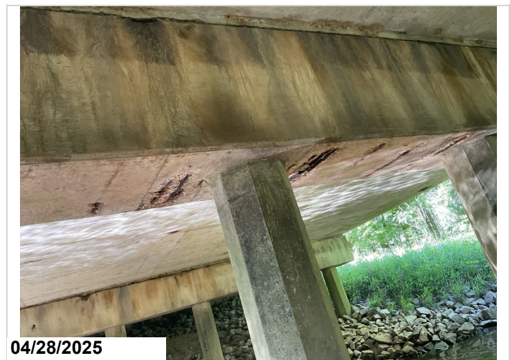
Cap Bent 3: Spalls with exposed rebar on bottom.
