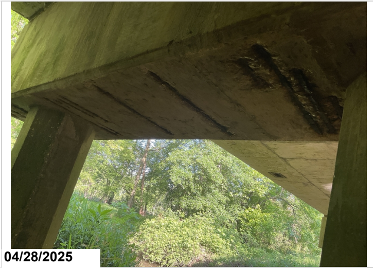
Cap Bent 2: Spalls with exposed rebar on bottom.
