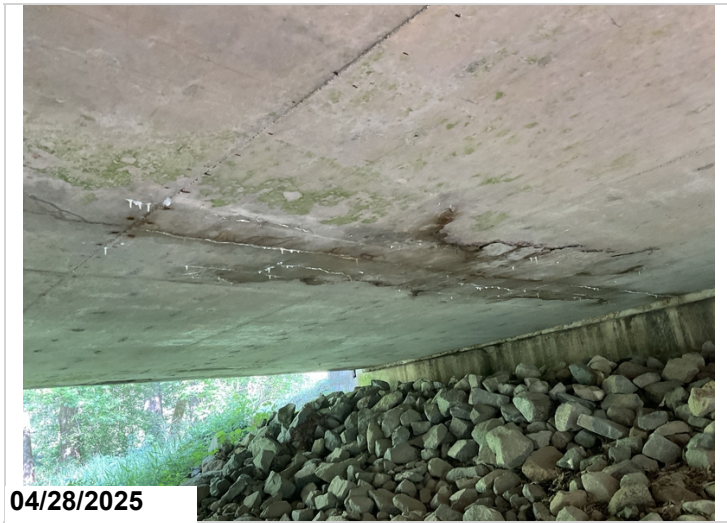
Undersurface Span 4: Large delamination with staining.
