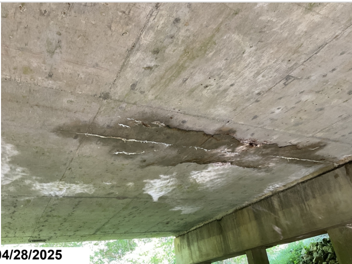
Undersurface Span 3: Large delamination with staining.
