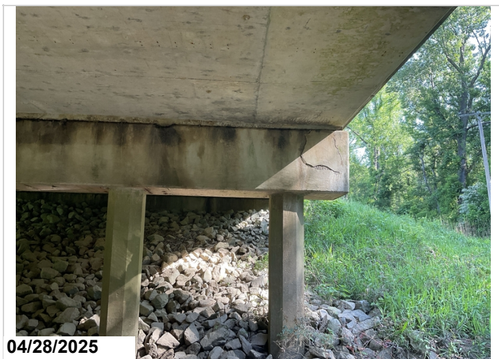
Cap Bent 4 Back: Large delamination on right end.
